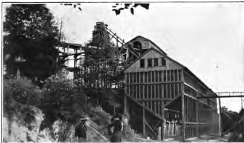
A. ABANDONED BUNKER OF THE ISSAQUAH COAL CO., AT ISSAQUAH, KING COUNTY.
